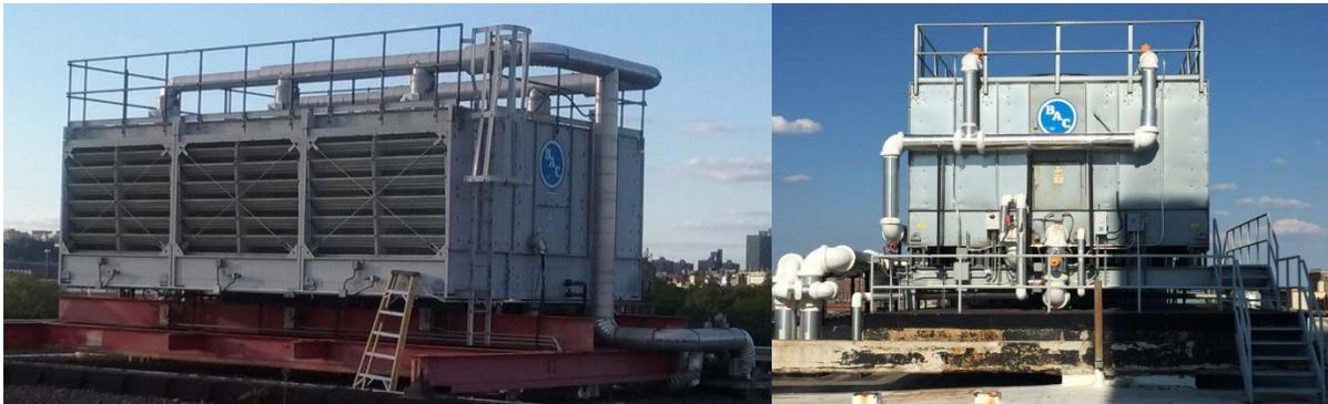
Some large cooling tower systems have more than one tower. Additionally, some cooling towers have more than one “cell” (sometimes called a “basin”). For example, an “eight-cell tower” is one cooling tower with eight cooling tower “cells.” As long as the different cells inside a cooling tower and the
